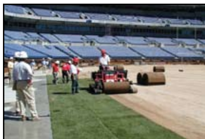
Example of laying sod on a football field. Photo: Ross Kurcab, CSFM
