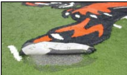
Installation of a special logo on a synthetic field. Photo: Darian Daily
