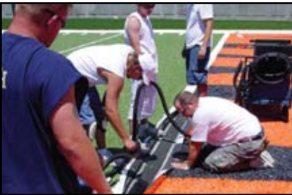
Seam construction on a synthetic field. Photo: Darian Daily
