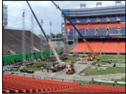
Set up for a concert showing field protective coverings. Photo: Ross Kurcab, CSFM
